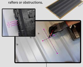
Mark the roof surface using desired penetration hole size tick marks. Mark the center on the north side of the lid. Connect three lines using a straight edge to determine the center for hole saw pilot bit.
