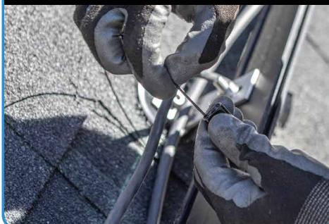
3. Turn cable 180° and insert through final open hole. Pull tight to lock.
